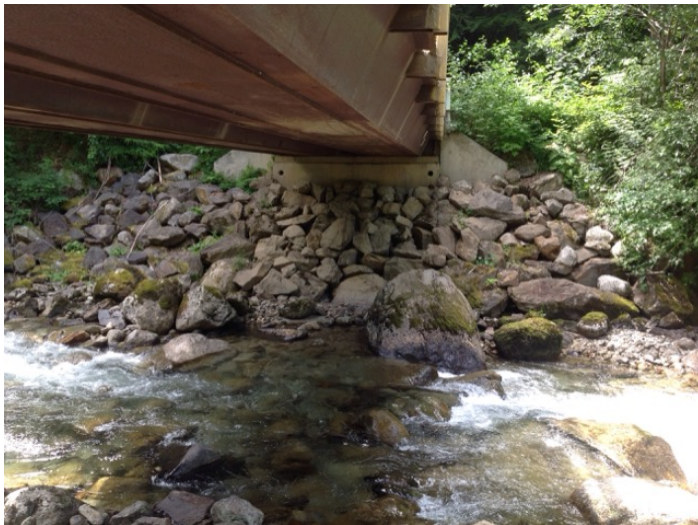
Left Bank Abutment when facing downstream
