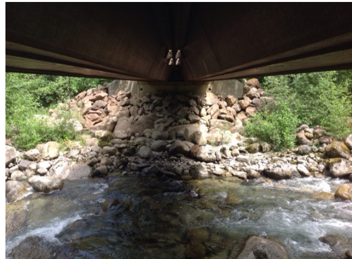
Right Bank Abutment when facing downstream
